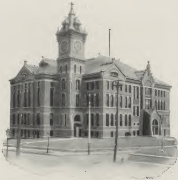
The Old Building
